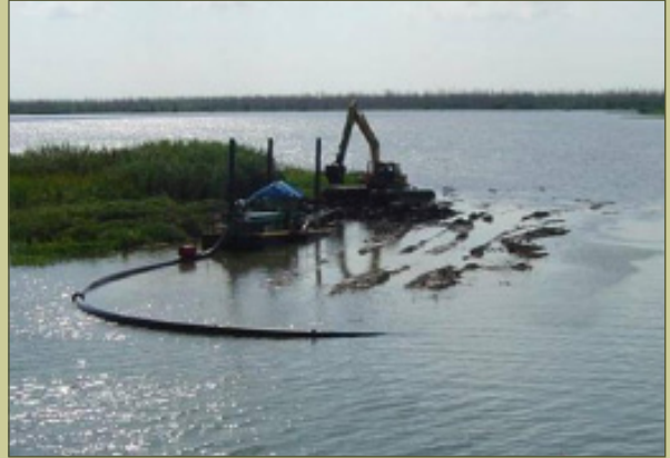
Ocean Energy, Inc. restoration site.
