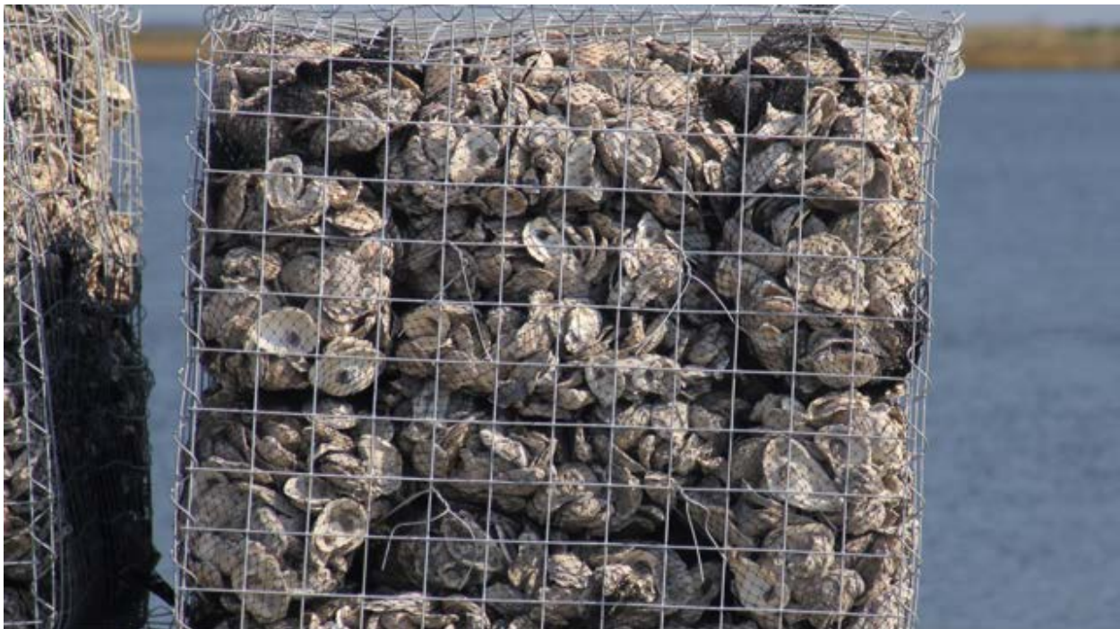
FIGURE 3-12. Gabion filled with oyster shell (Source: https://www.brproud.com/news/fighting-coastal-erosion-a-louisiana-tribe-banks-on-oyster-shells/ ).
