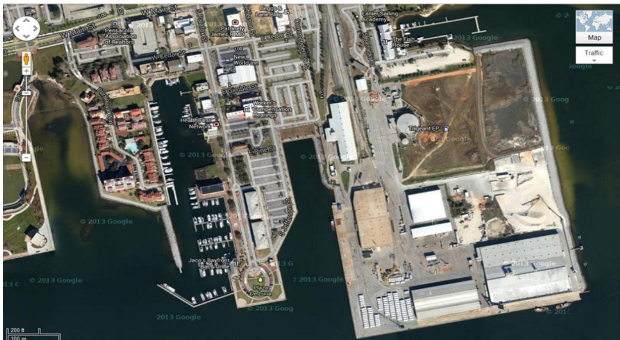
Figure 12-21. City of Pensacola connected actions approximate area next to Plaza de Luna facility where parking lot, landing, ramp, dock and passenger queuing area would be.
