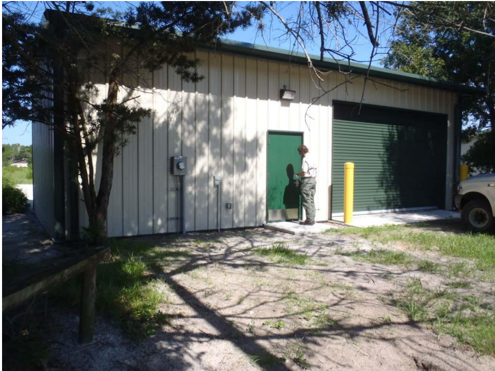
Figure 12-24. Support shop facility example.
