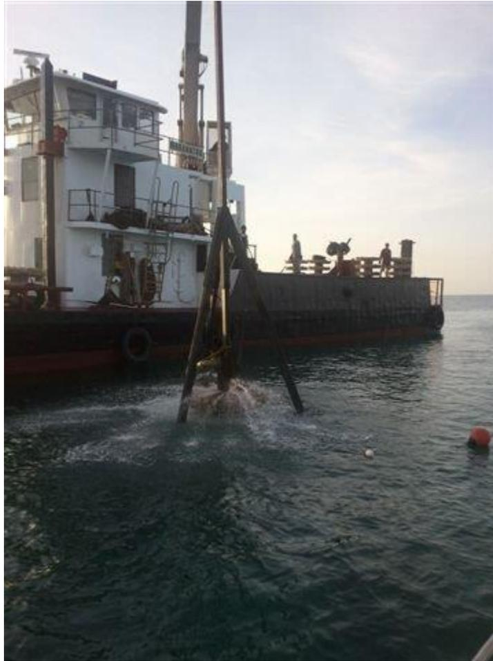
**Figure 12-36.** Example of a disk-type reef being placed with seawater being pumped through its central pipe
