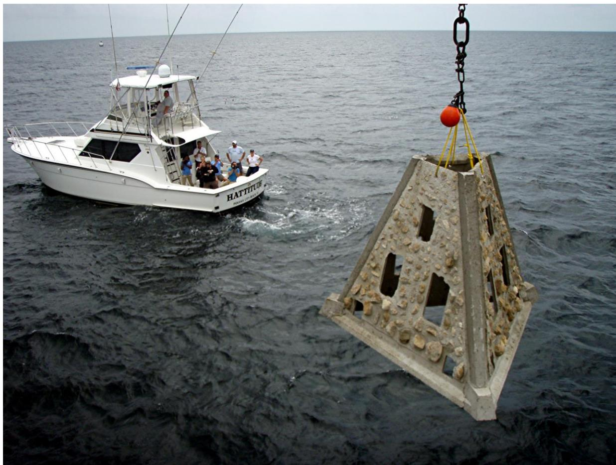
**Figure 12-34.** Example of a pyramid type reef being deployed.
