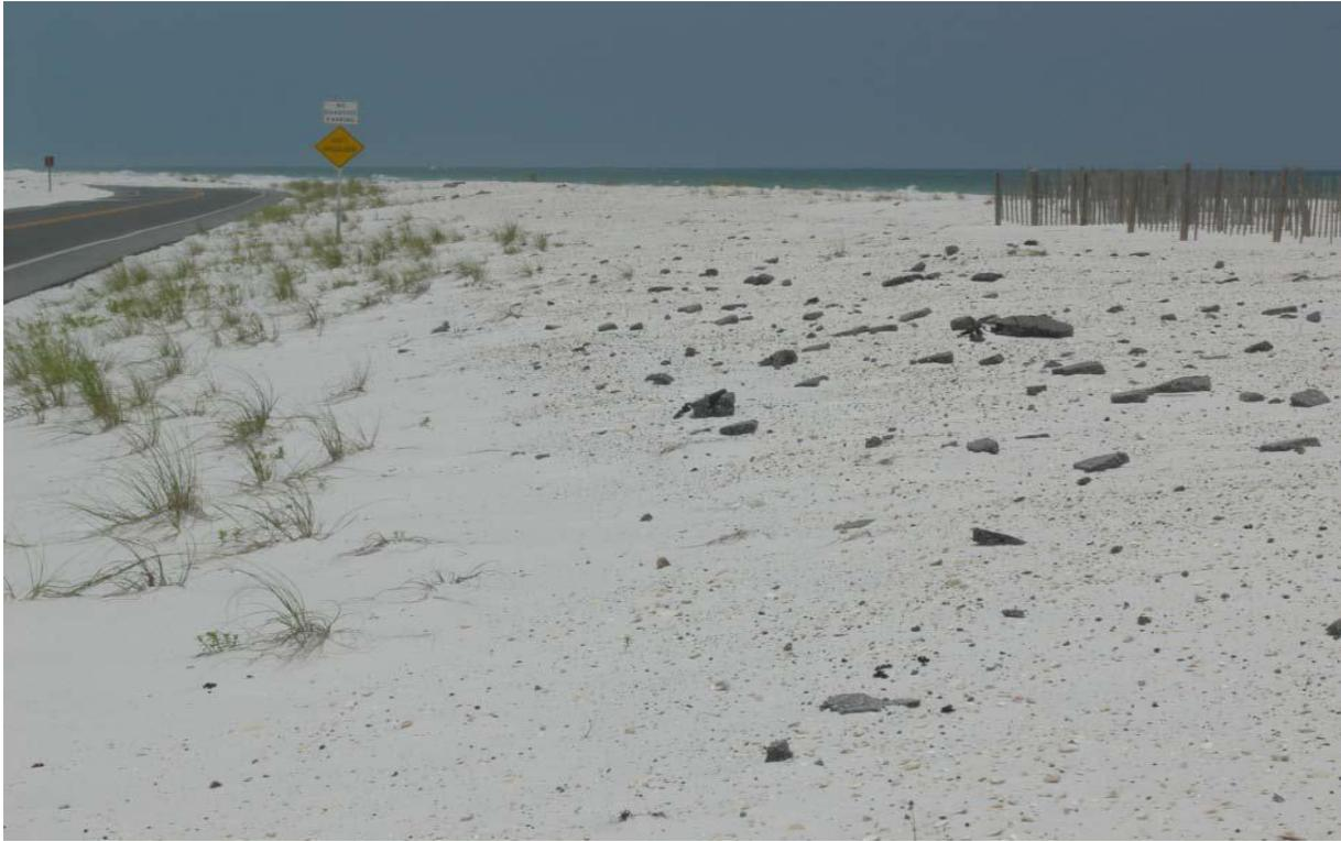
Figure 12-3. Asphalt fragments and road-base materials.
