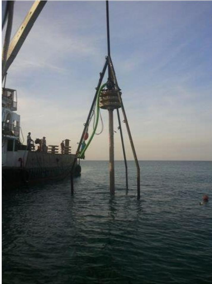
**Figure 12-35.** Example of a disk-type reef being deployed while still in its supporting tripod.
