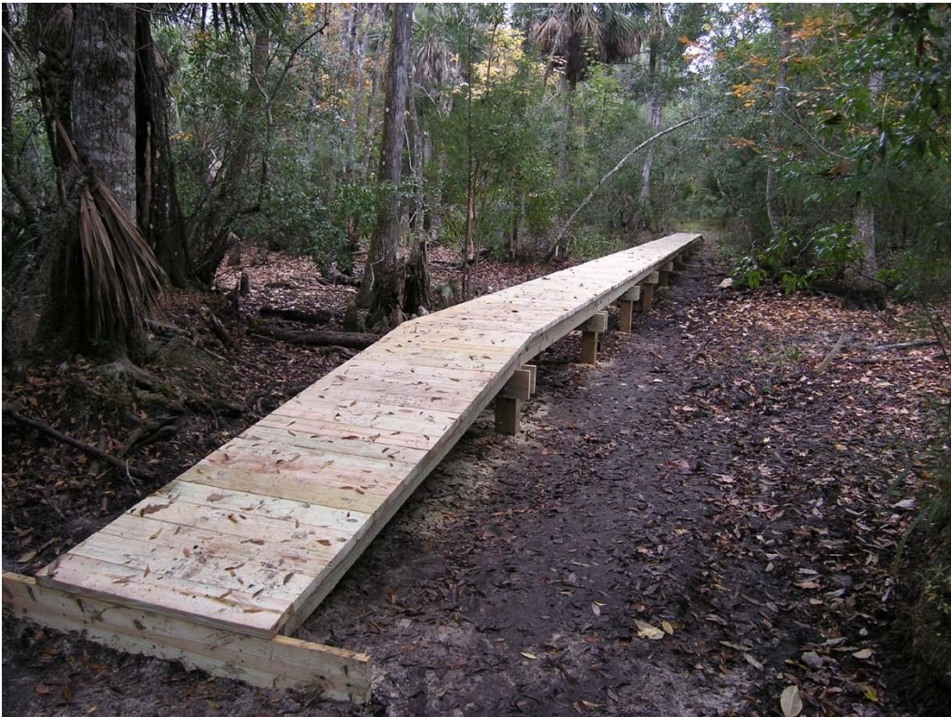
Figure 12-38. Elevated Walkway Example.
