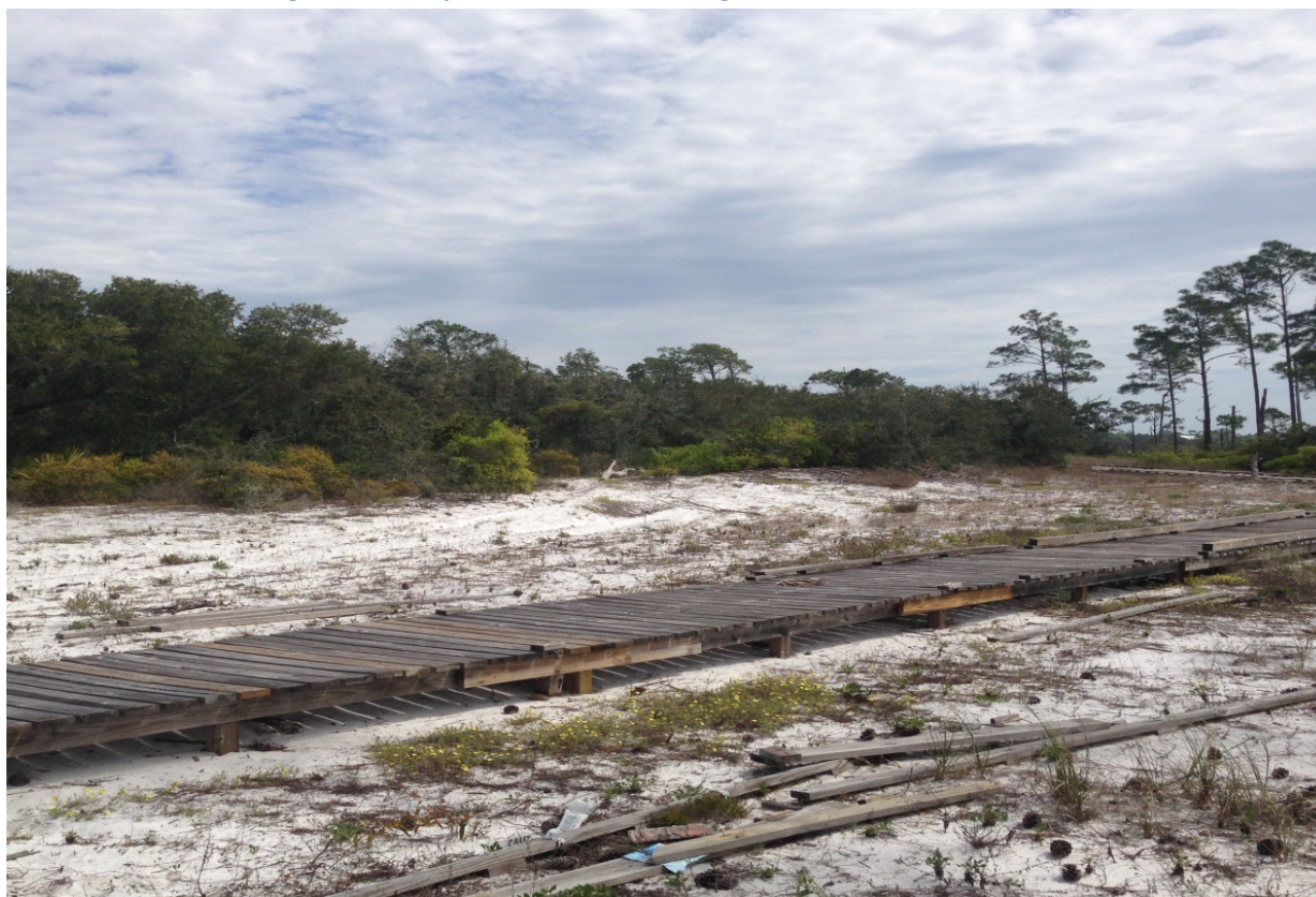
Figure 8-4. A portion of the existing Jeff Friend Trail boardwalk
