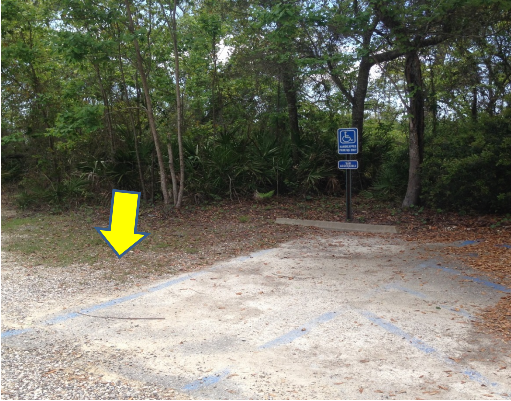
Figure 8-3. Existing handicap parking area (yellow arrow) that is to be widened
