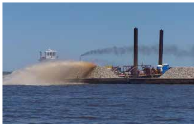
A barge deploys oyster shells to restore subtidal oyster reefs in St. Louis Bay, Mississippi.
