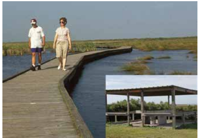
This marsh boardwalk and fish cleaning station are similar to structures in the Sea Rim State Park Improvements project in Texas.
