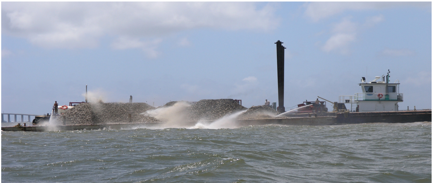
Cultch Planting with Water Cannon to Efficiently Spread Cultch Material
