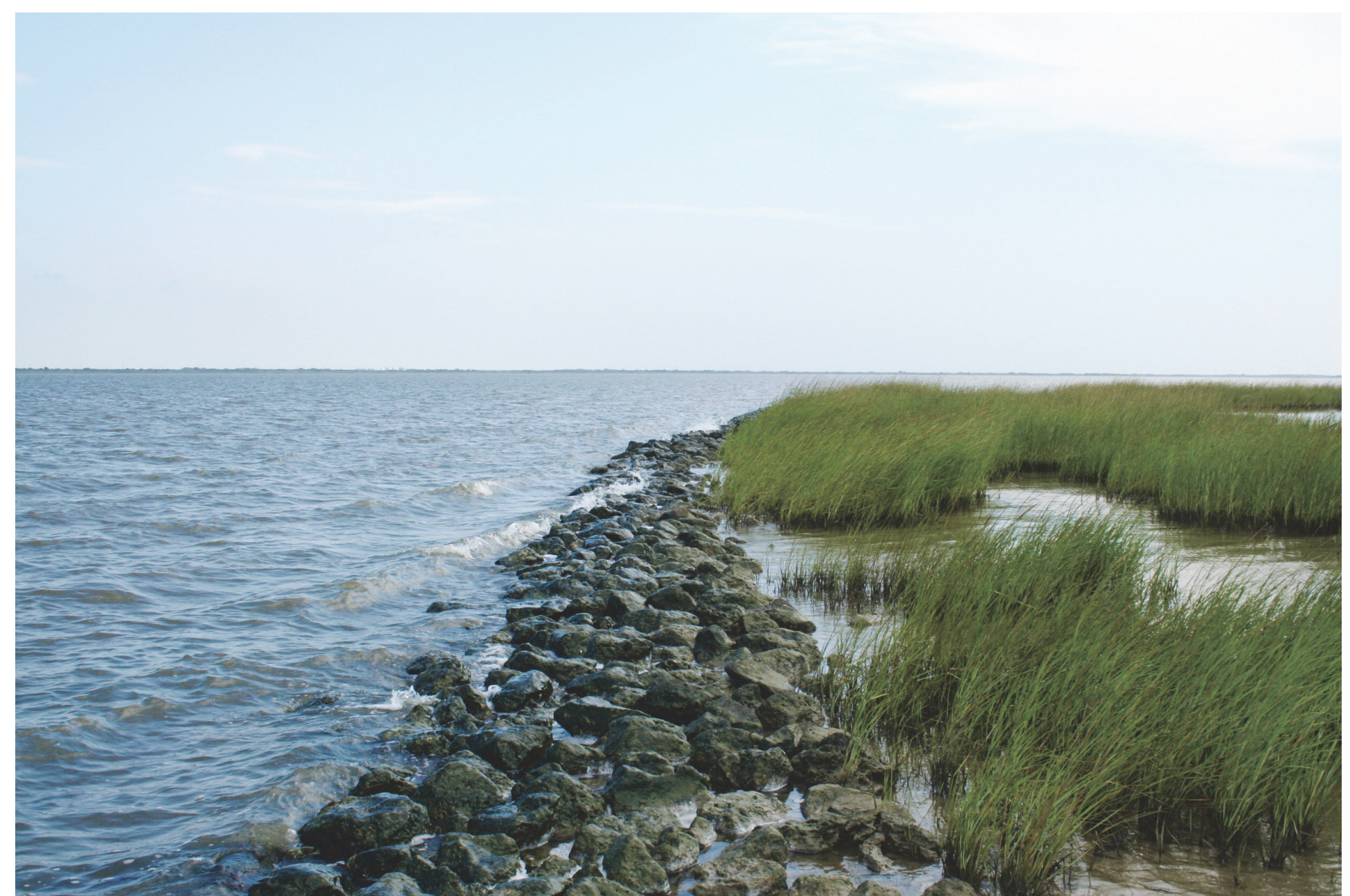
Powderhorn Lake, Indianola, TX Example of a living shoreline using sills technique
