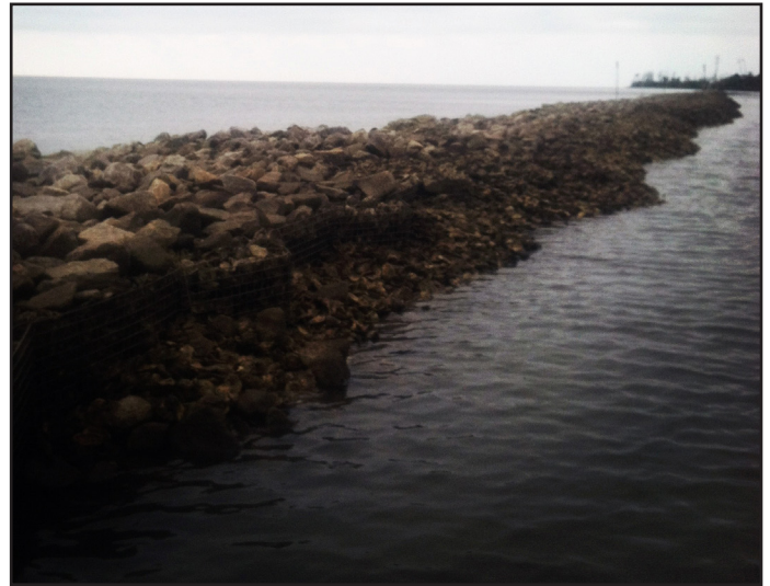
Living Shoreline Breakwater at low tide at Swift Tract, Alabama. Photo courtesy of The Nature Conservancy - Mary Kate Brown.
